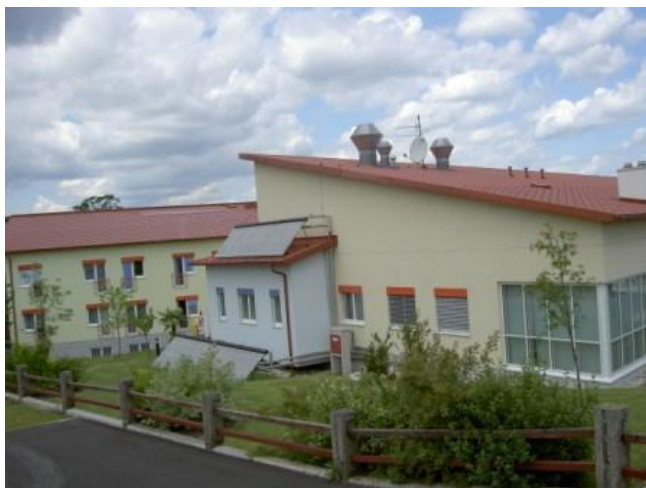
Outdoor shot of nursing home Schrems The heated gross floor area amounts 5.294 sqm.
