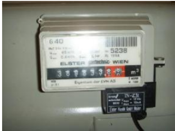
natural gas counter with reed relays
